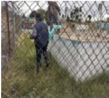
Rebombeo Constanica I
